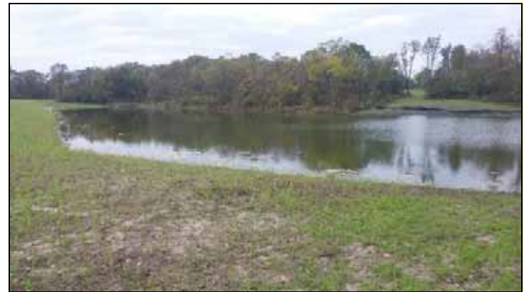
Pond Structure stabilizing large gully depositing sediment into Big Creek Lake
